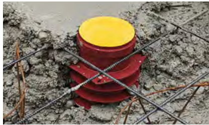
Add concrete and vibrate
