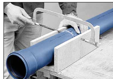
Cutting to length with fine-toothed saw
