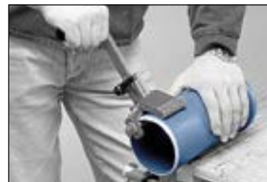
Bevelling with a bevelling tool
