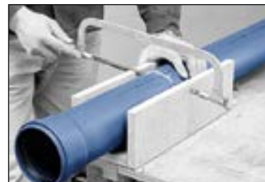
Cutting to length with fine-toothed saw
